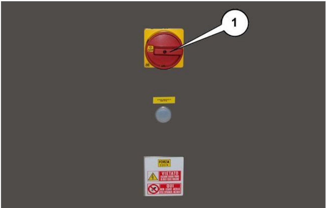
Figure 3- 3 - Location of the main switch (1)
